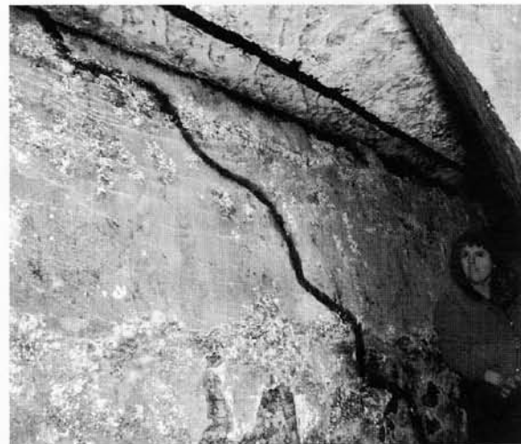
Figure 26. Room 5, left wall.
